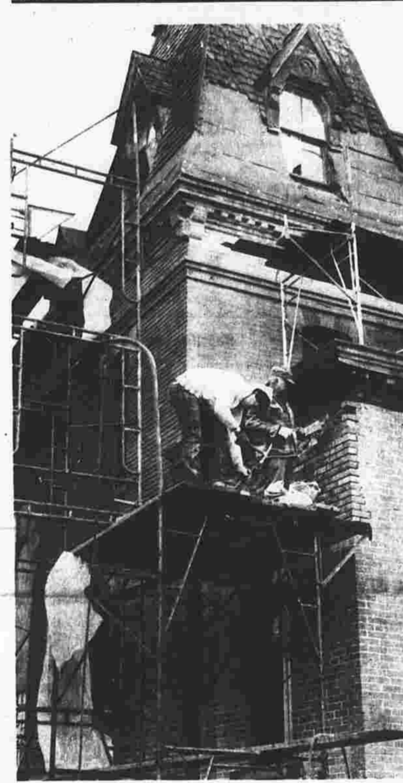
Renovating history Bruce Bates, left, of Manchester, and Arnold Holmes, of Glassbury, replace bricks and repoint brickwork at the front of Cheney Hall (above and at right). They are employed by Alma Construction of Vernon, a subcontractor on the $243,000 Cheney Hall exterior-renovation project. The general contractor for the exterior renovations, which should be completed by spring, is the Metro Building Co. of Manchester. A spokesman for Metro said about 75 percent of the brickwork is completed. Top right, wood burning in a barrel heats up bricks before they are laid.
