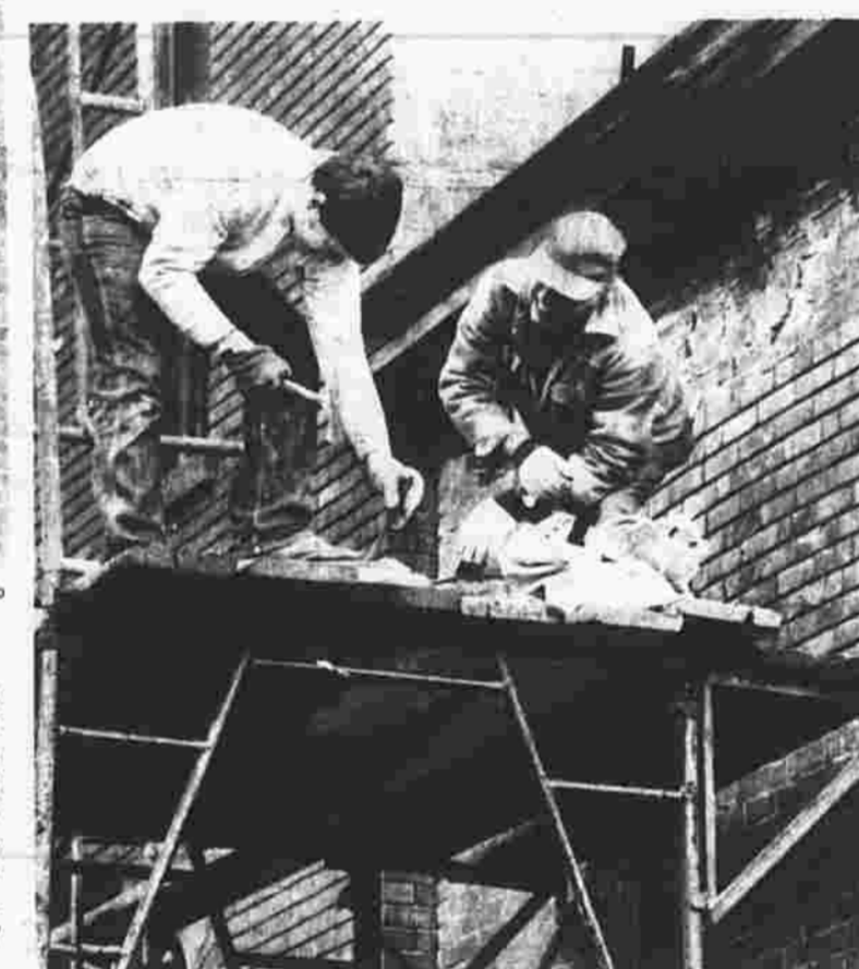
Renovating history Bruce Bates, left, of Manchester, and Arnold Holmes, of Glassbury, replace bricks and repoint brickwork at the front of Cheney Hall (above and at right). They are employed by Alma Construction of Vernon, a subcontractor on the $243,000 Cheney Hall exterior-renovation project. The general contractor for the exterior renovations, which should be completed by spring, is the Metro Building Co. of Manchester. A spokesman for Metro said about 75 percent of the brickwork is completed. Top right, wood burning in a barrel heats up bricks before they are laid.
